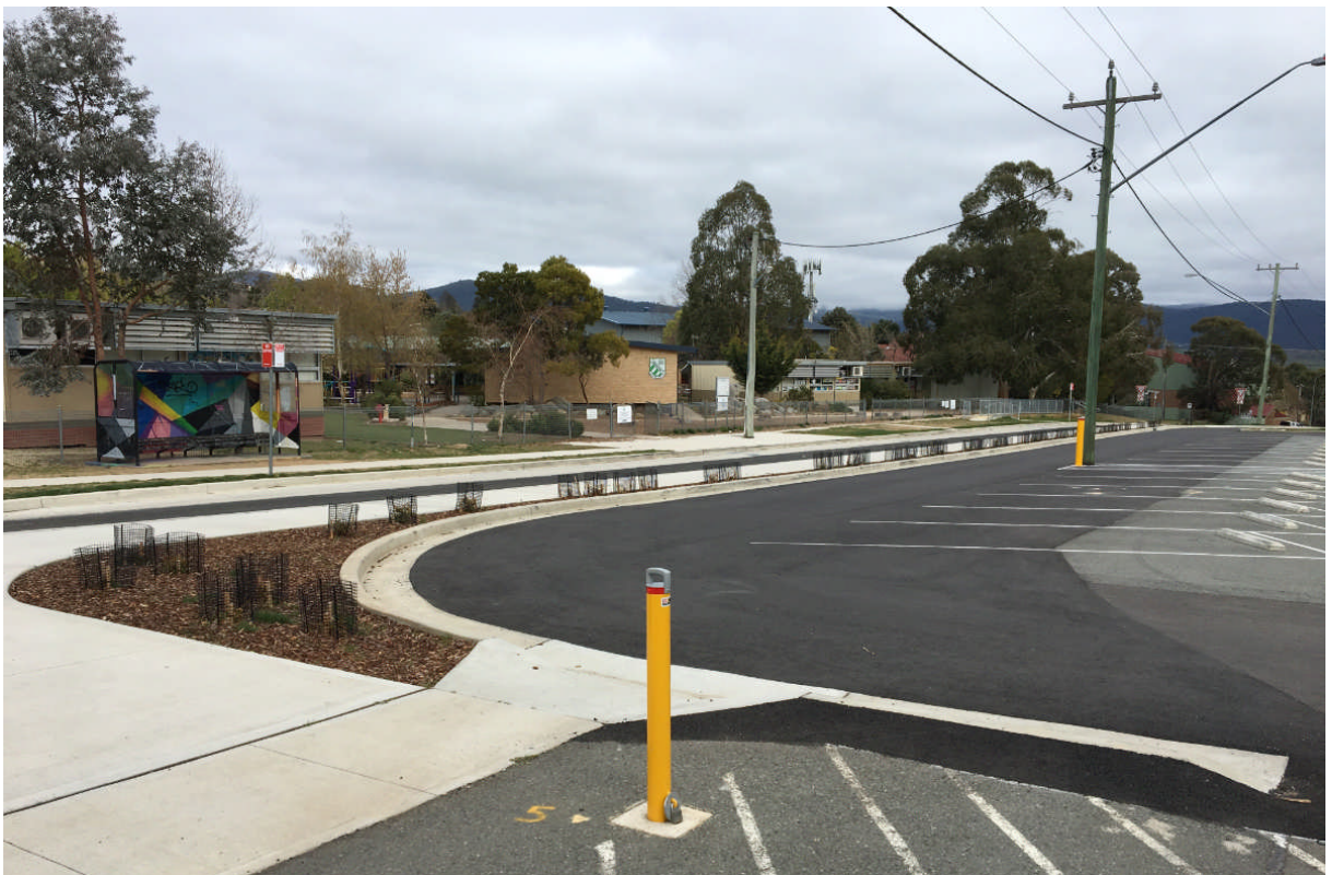
View from Kalkite Street Carpark to the Primary School main gate and bus set down area
