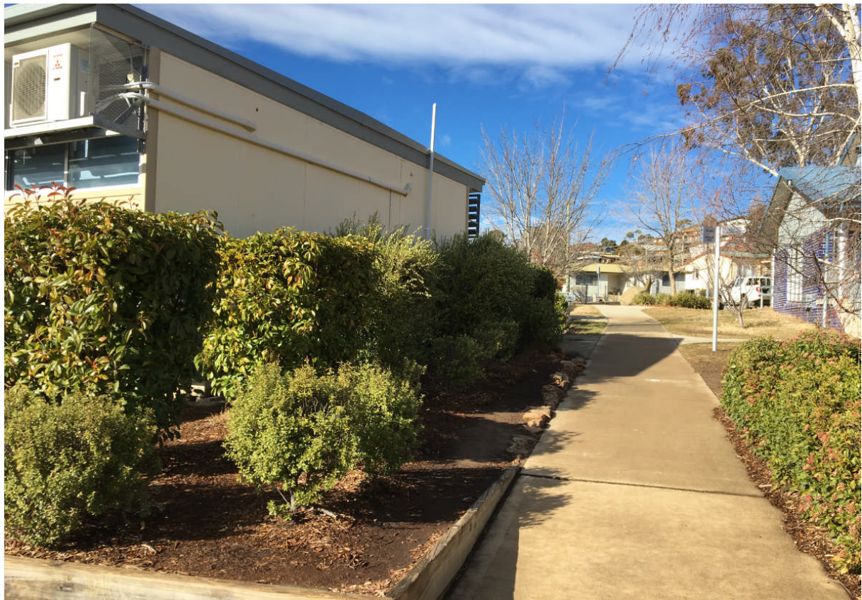
Looking South to the existing Park Road entrance with demountable building to be removed in the foreground.
