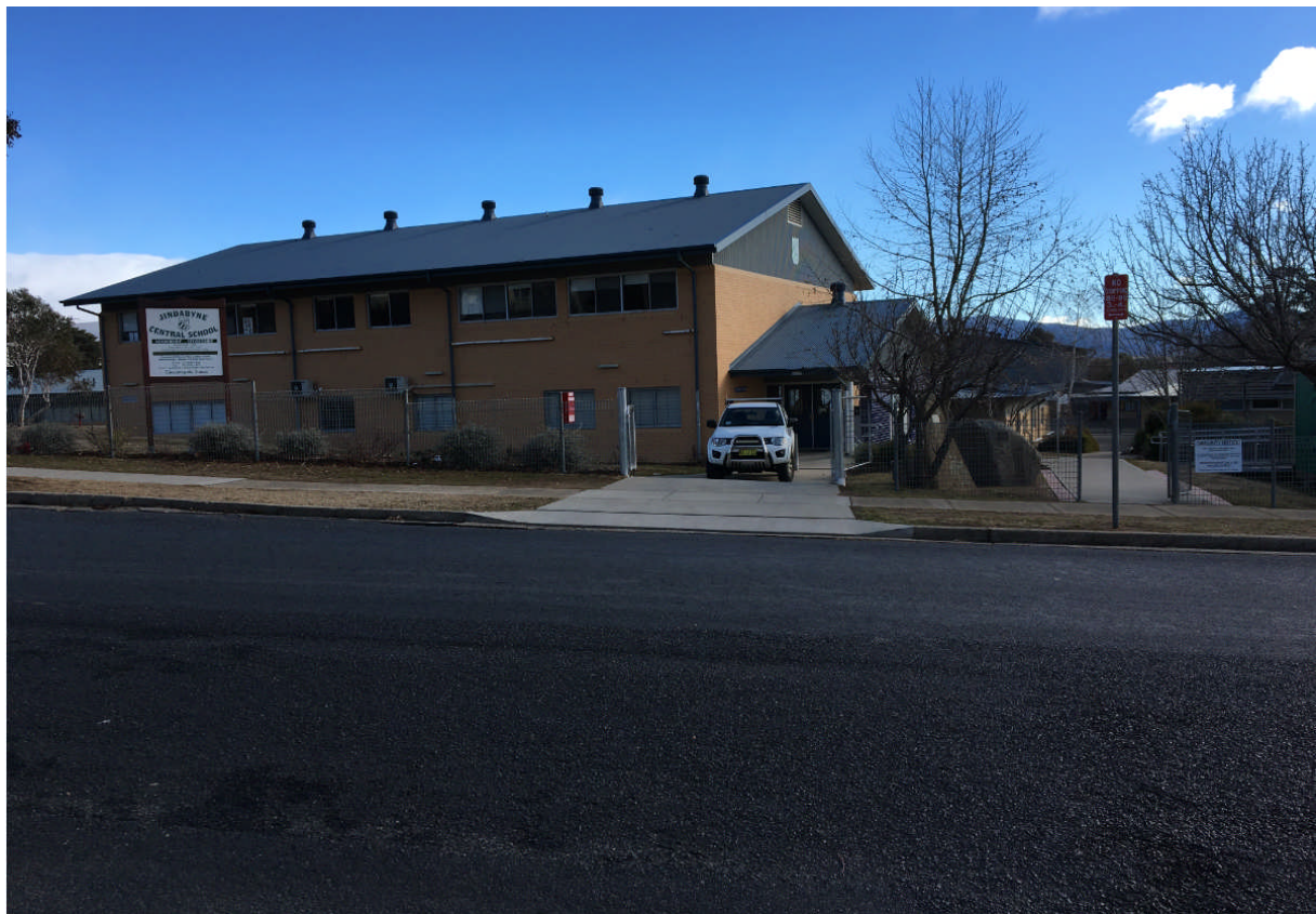
Existing administration building when viewed from Park Road
