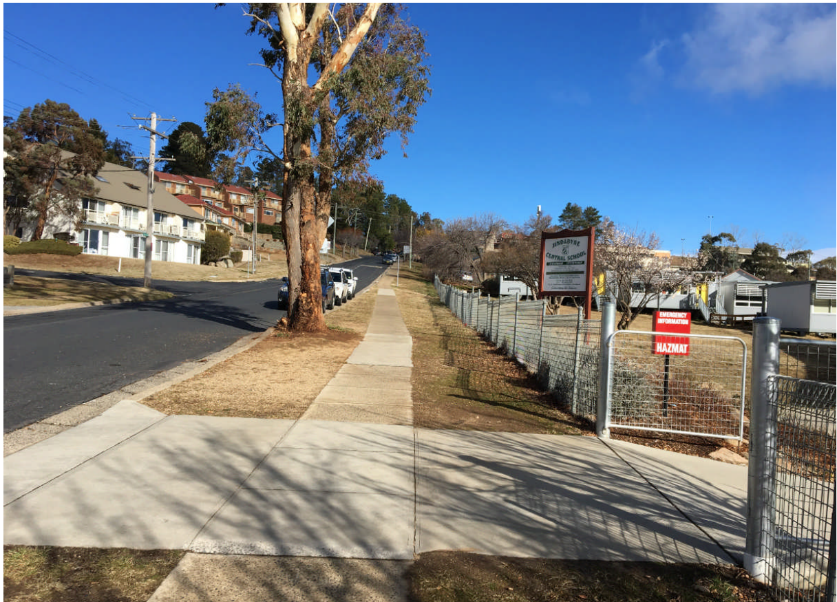
View looking west up Park Road with current vehicular access to the Administration building in the foreground. This access will be closed and moved further west for the new carparking area.
