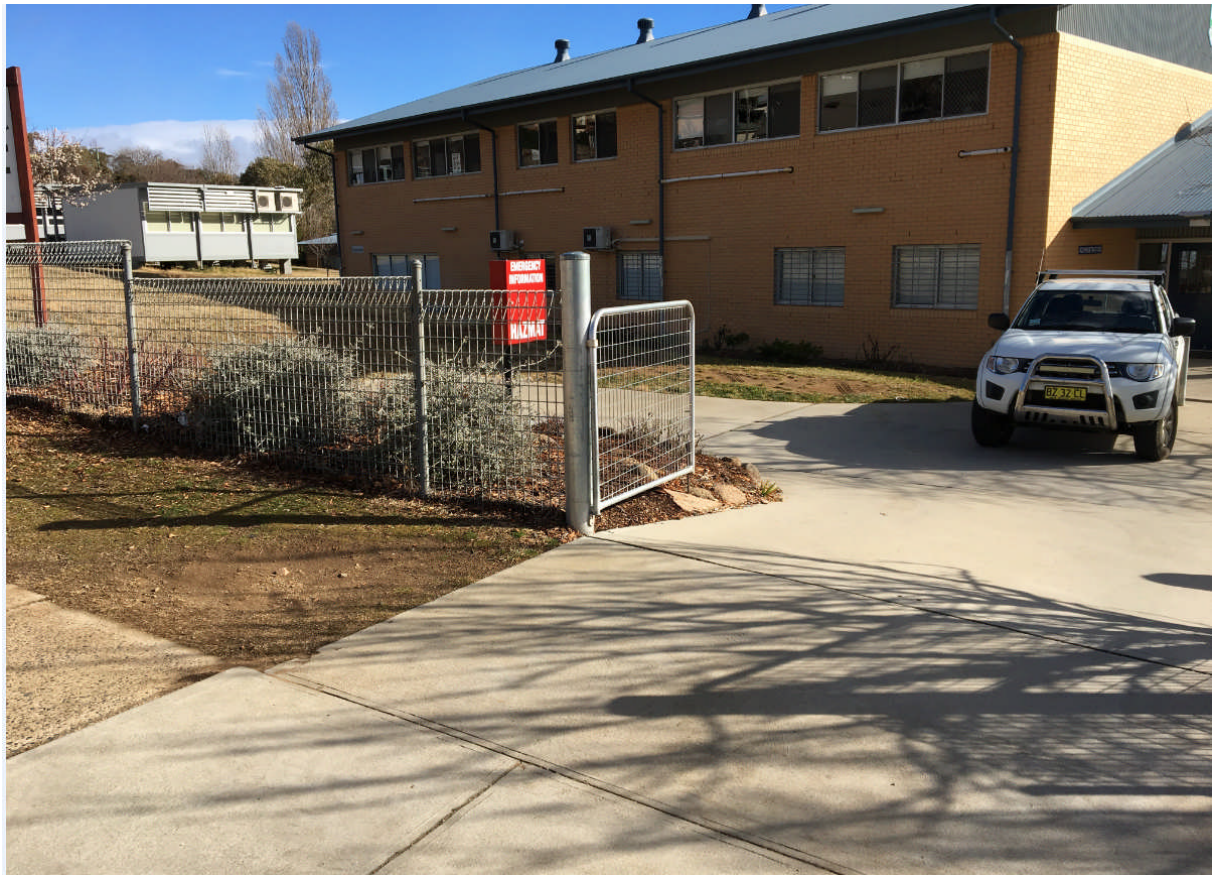
Existing vehicular entrance to administration building
